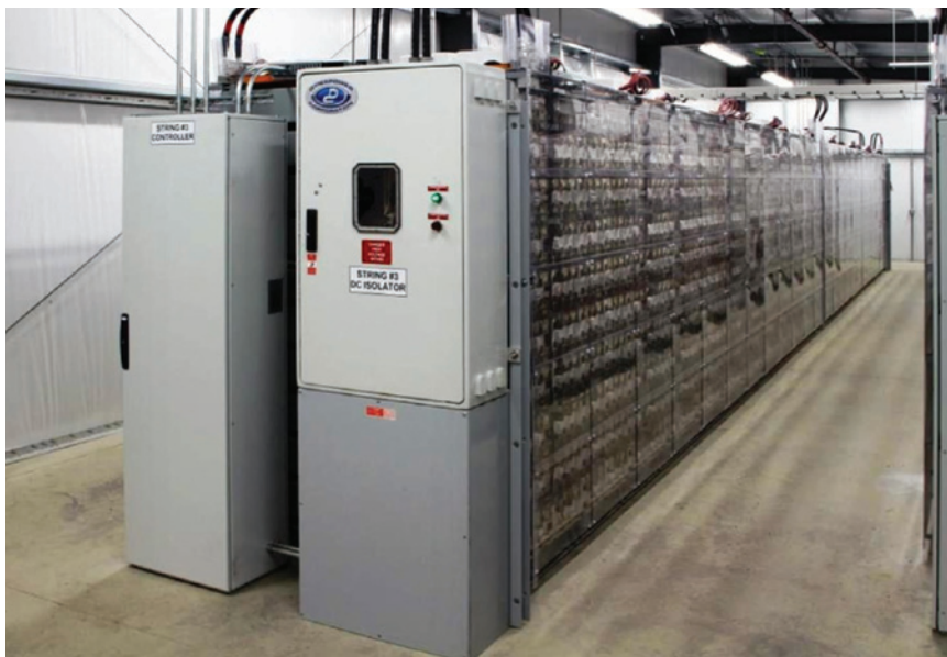
Lead-based Ultrabattery® used for frequency regulation at Lyon Station, Pennsylvania
